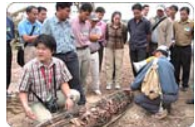
Figure 3. Laos—Technical cooperation on riverbank protection works
