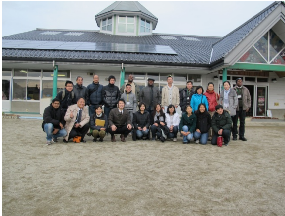
The solar panel on the roofs of Kanae Mitsuba Nursery
