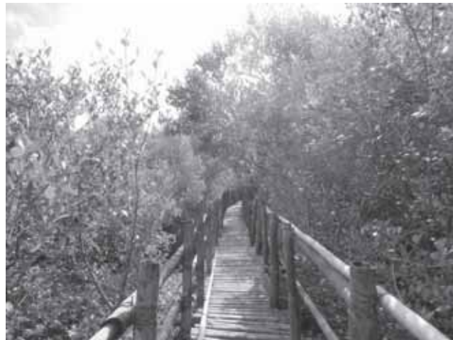
Figure 4: A bridge used for monitoring and eco-tours in the Mangrove forest in Balarang
