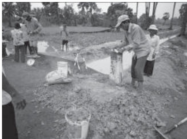
Figure 4: Admixture of soil-cement component material
